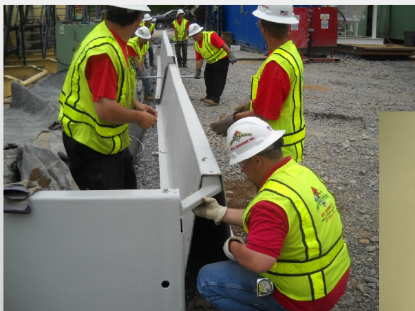
Rigid barrier is liquid proof with overlapping seam design
