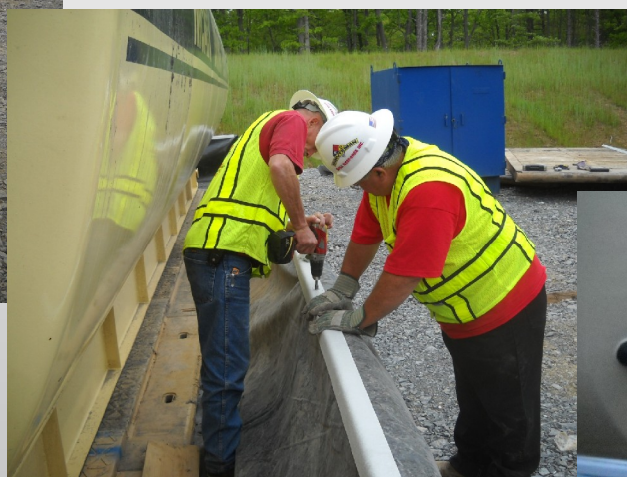
Heavy 30mm liner, held in tension, and secured with barrier cap
